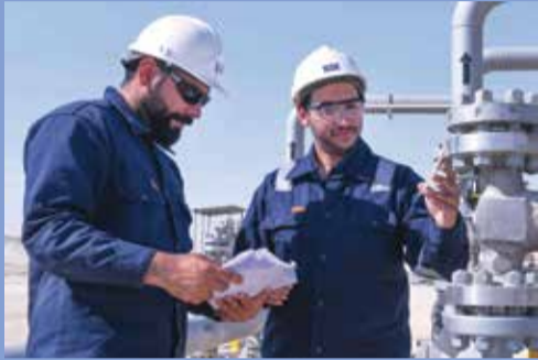
From left, crew members Majed M. Al Shammari, mechanical piping quality control inspector, and Mustafa S. Al-Mulla, mechanical engineer, review the quality checklist for the oil well infrastructure. To ensure quality, the crew members underwent additional extensive preparation, including a six-month training program overseen by certified personnel at the contractor's premises, and they had to be certified by Saudi Aramco's Inspection Department in their respective fields.
