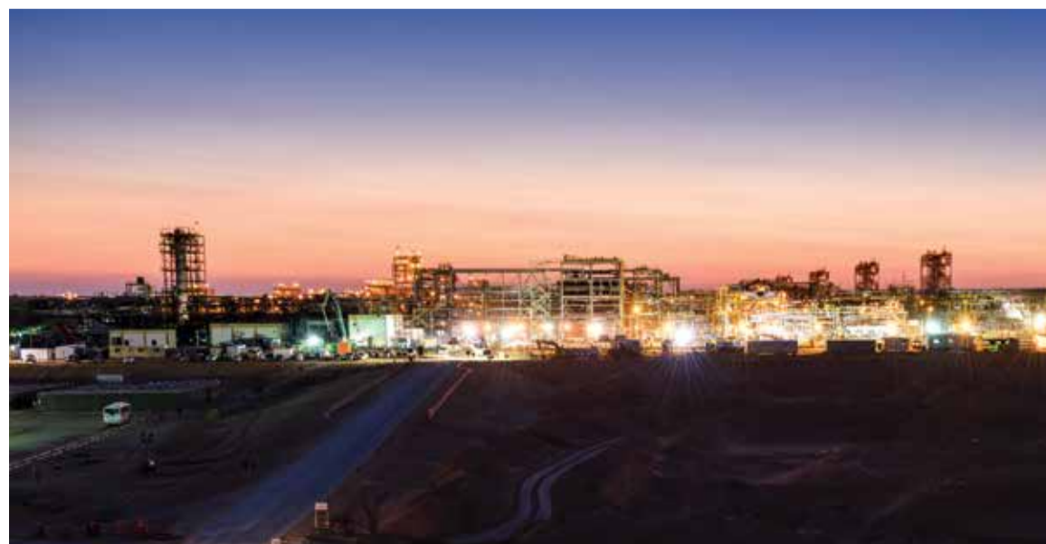
Officials recognized the major completion milestone of the first oil for the Khurais Arabian Light Crude Oil Increment program.
