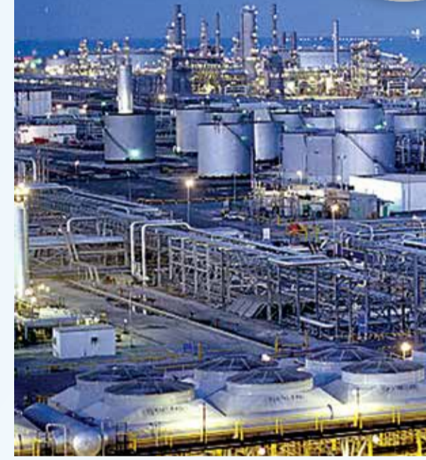
Drone-mounted cameras are used to monitor and measure
