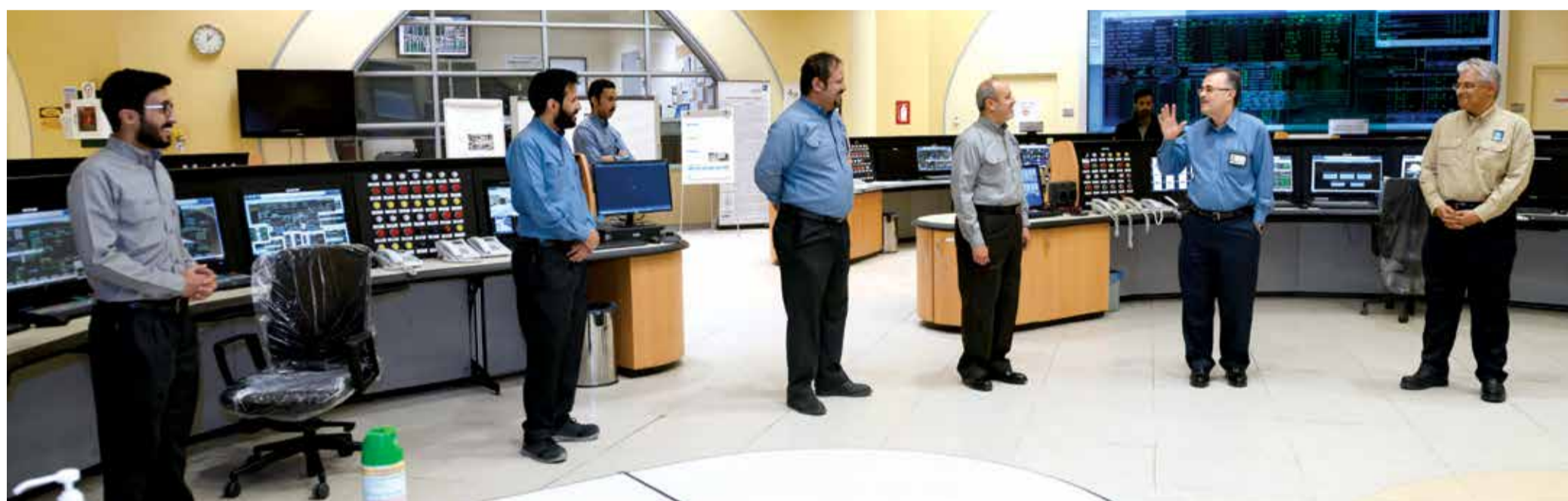
Amin Nasser is joined by other members of management during a recent visit to control facilities in Khurais. The president and CEO noted that the same resolve shown by employees in the face of last year's attacks on our facilities is the same he is seeing now by Aramco's companywide as they respond to the threat of COVID-19. "Our people across company facilities are highly motivated to succeed now more than ever," he said.
