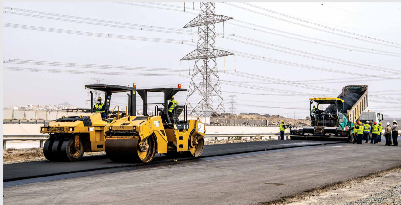
A new concept introduced by Saudi Aramco is looking to transform waste tires into a resource. The innovative concept is to turn crumb rubber from the tires into a form of asphalt used in laying and maintaining roads, such as the road construction project at the North Jiddah Bulk Plant Expansion Project. (Photo: Ahmad El Itani/MPD)
