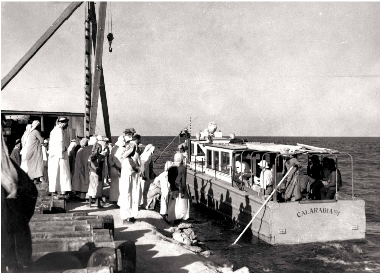
Residents board a boat for Bahrain in the late 1930s, long before the causeway provided an automobile route to the island. Floyd Ohliger, a prominent figure in Aramco history, supervised the construction of the al-Khobar pier, the very first of its kind. The boat Calarabia departed regularly to Bahrain from the pier. Photo: Max Steinke
