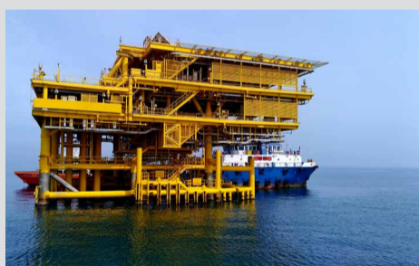
The "SSS" offshore wellhead comes in two design types — electrified and nonelectrified — and their electrical cable trays, junction boxes, signage and posts, sunshades, wind socks, and utility piping abide by Aramco's requirement for the inclusion of nonmetallic materials.
