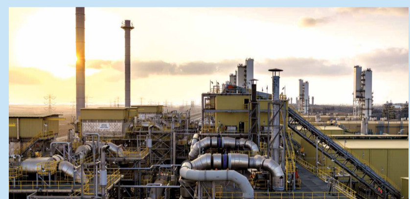
Jazan's soot ash removal unit sits within the integrated gasification combined cycle power plant.
