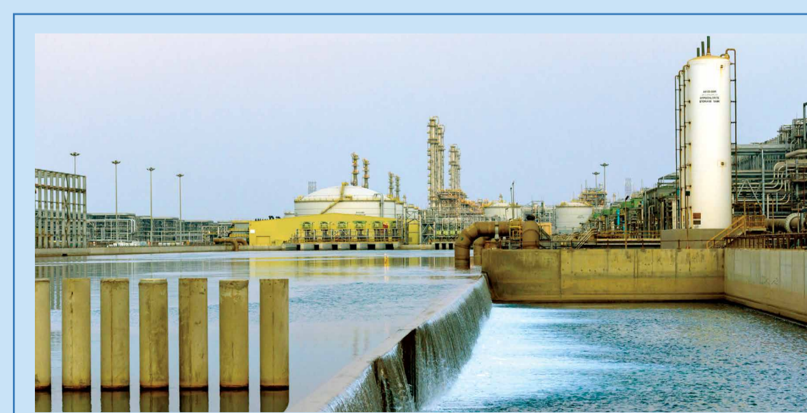
Jazan plant's seawater lagoon.
