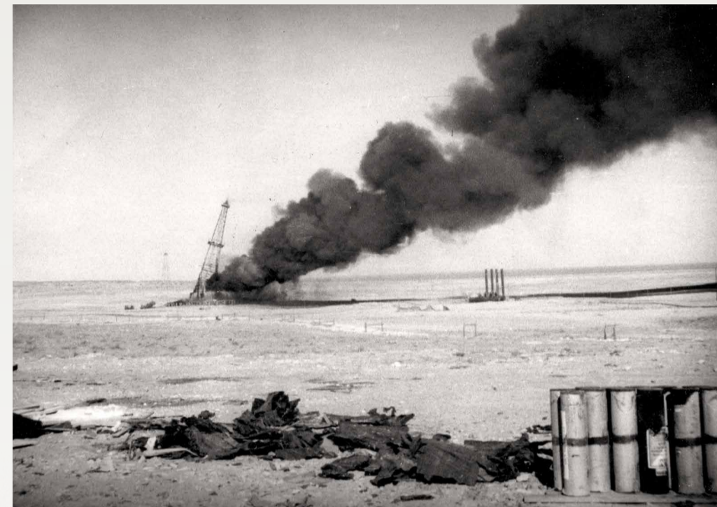
The fire at Dammam Well-12 on July 8, 1939, burned so hot that the 41-meter-high derrick collapsed after roughly 10 minutes.
