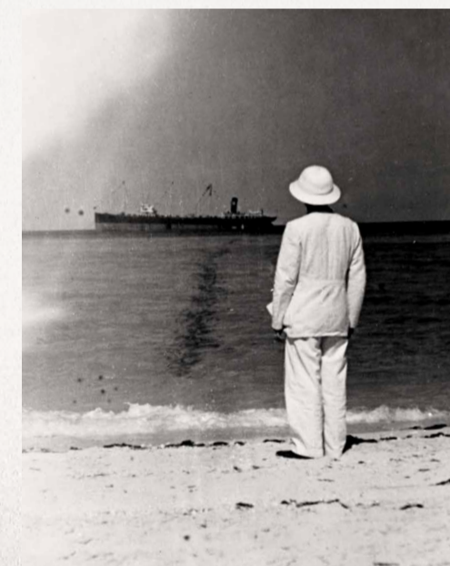
On May 1, 1939, a submerged pipeline delivers crude oil from Ras Tanura to the tanker D.G. Scofield, which is moored about one kilometer offshore.
