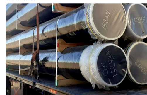
Left and above, installation of the RTR pipes. Below, RTR pipes being transported to the work site.
