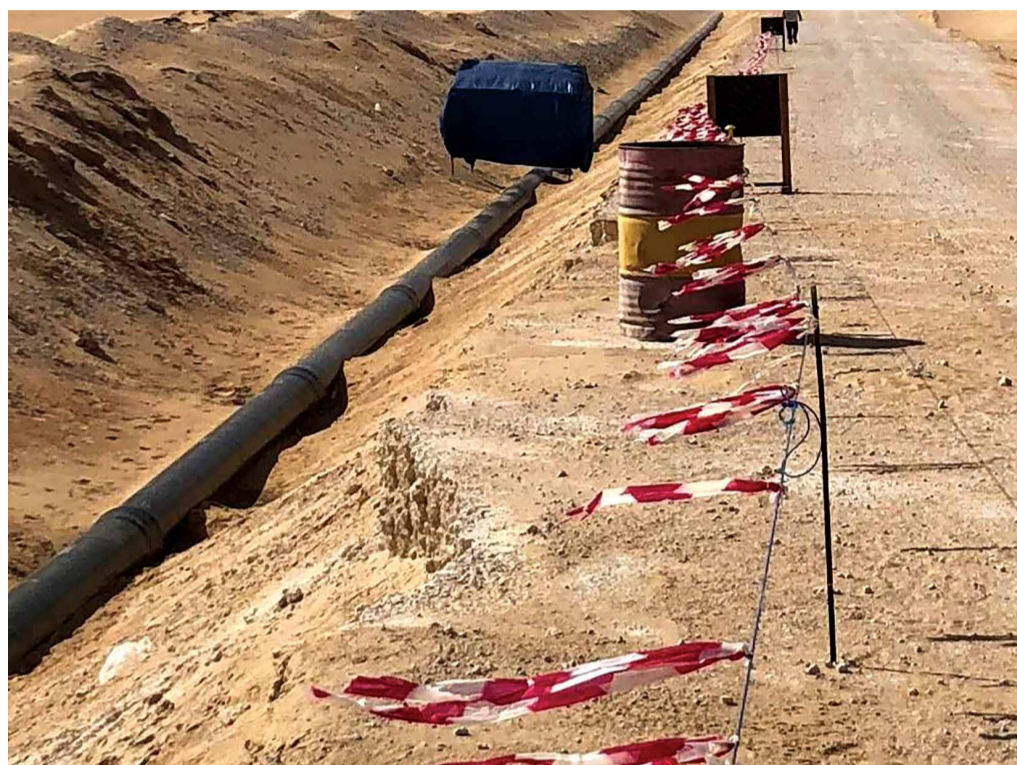
Left and above, installation of the RTR pipes. Below, RTR pipes being transported to the work site.
