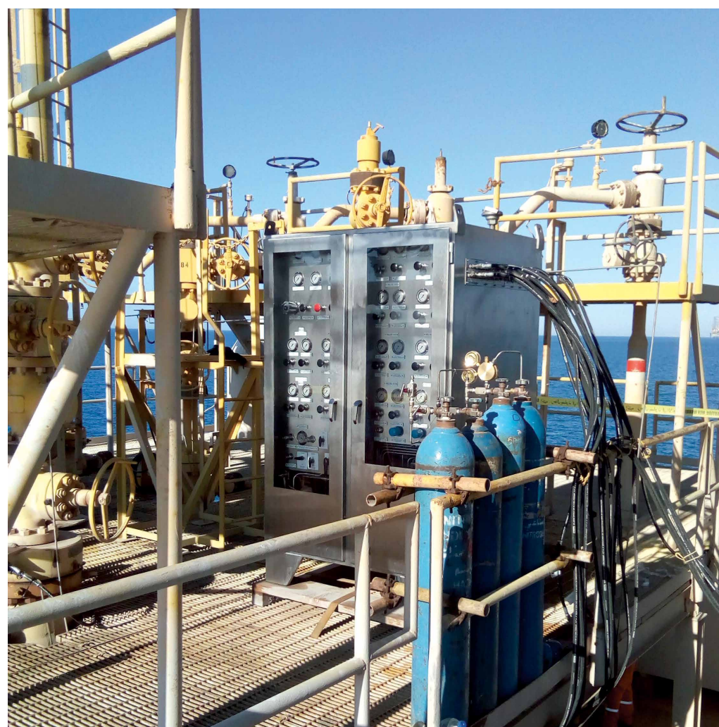
The successful deployment of a portable emergency shutdown system in the Zuluf oil field.
