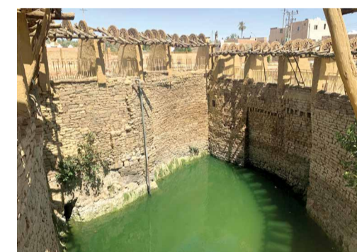
Hadaj Well can water 100 camels simultaneously. The well perimeter is 65 meters, and its depth is around 12 meters.
