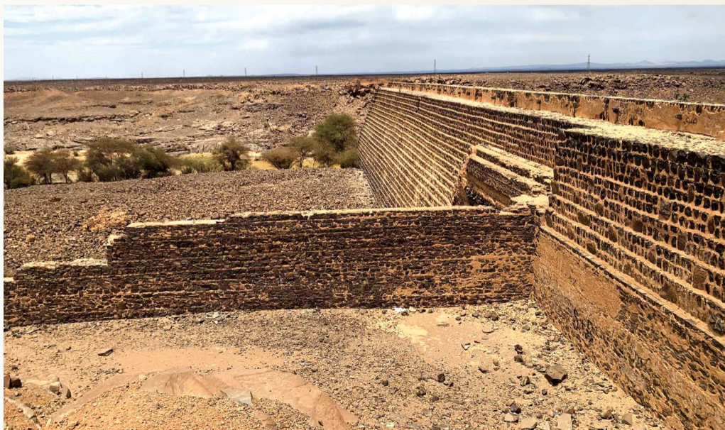
Al Bint Dam is mostly in a good condition, even though approximately one-third of the dam has fallen. Some claim that it was built in the early Islamic era, and others say it was constructed in the third century B.C.
