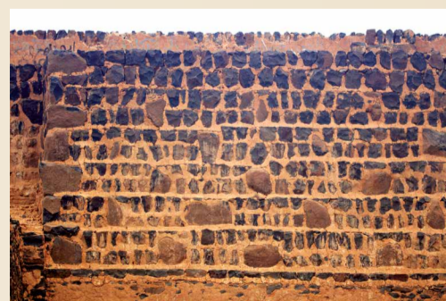
The texture and quality of the mortar used in Al Bint Dam is similar to Marib Dam, which was built by the Sabaeen Kingdom. Interestingly, local tradition says that the dam was built by a prince from Yemen as a dowry for a girl, i.e., the name.
