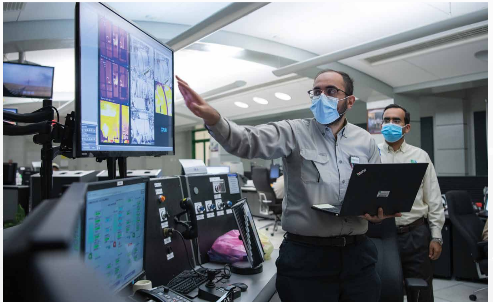
Working with technology makes for a lower carbon, more efficient, and safer operation, and in real-time, process engineer Turkey S. Alshuhail and operations shift superintendent Bdah F. Hajri examine thermal images monitoring the 1,200 degree Celsius metal skin temperature of Shedgum's sulfur recovery plant's refractory-lined reaction furnace to proactively identify any defects or hot spots requiring immediate isolation and repair.
