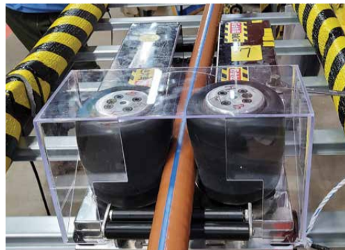
The new electrical cable pulling technology will be utilized in GOSP-4.
