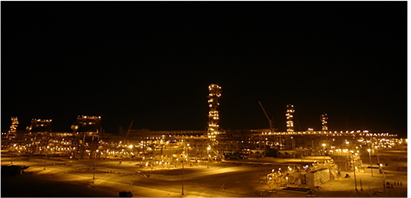
Hawiyah NGL Plant (Photo source : HNGLPD Electronic Gallery)
